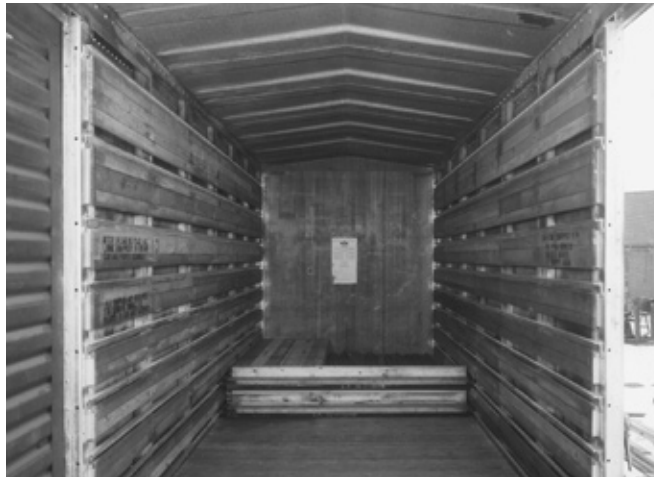
(Left, above) Among the most important innovations which began to be installed in box cars in the 1950s was the crossbar loader. The one shown here is a "9-belt" model, which refers to the horizontal angles or belt rails to which crossbeams or crossbars could be attached to divide and restrain the load. Other models with varying numbers of belts were also used. Stacked on the floor are wood-metal composite crossbars. In later years, these were usually all metal. The pioneer in this field was the Evans Products Company, whose loader installation is shown here. An example of one of these loaders in use is shown at right. (Southern Pacific photo, SUL)
